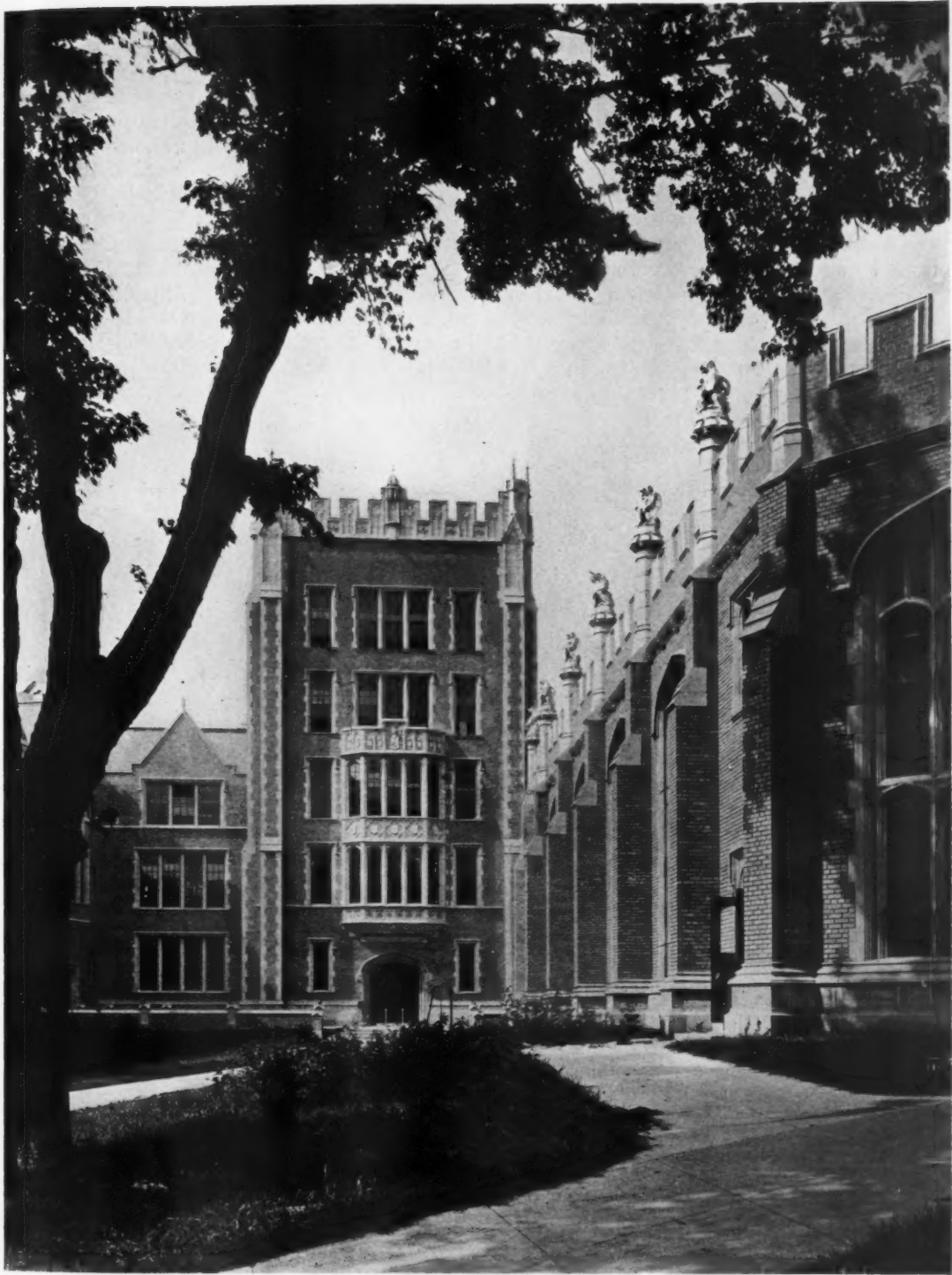
FLUSHING HIGH SCHOOL, FLUSHING, L. I., NEW YORK CITY
