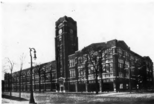
A MANUFACTURING BUILDING IN CHICAGO
