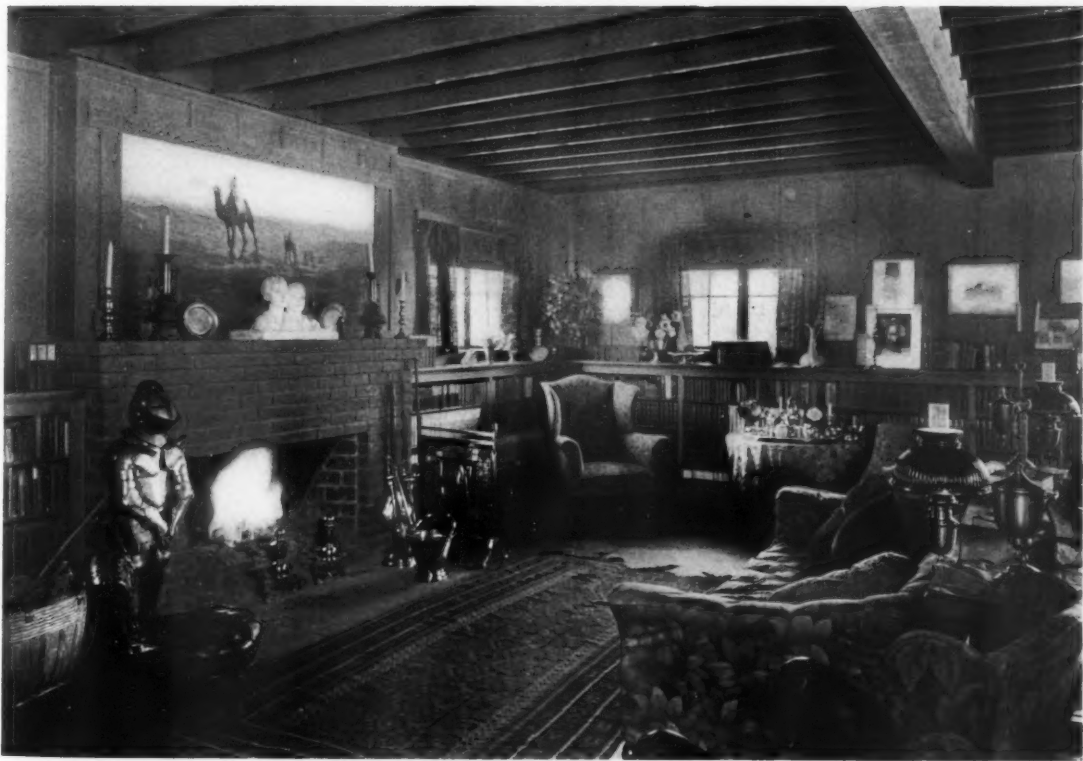
HOUSE OF PIERRE E. LETCHWORTH, ESQ., COVINA, CAL.
