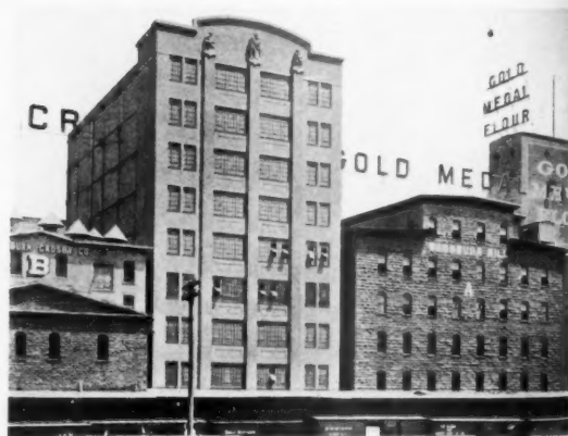
MILL ARCHITECTURE—OLD AND NEW—1880-1915
