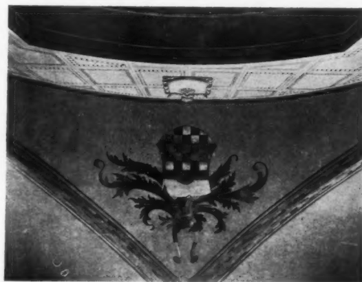
DETAIL OF GRILL ROOM CEILING
