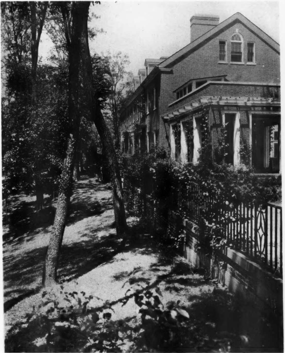
VIEW ALONG TERRACE FRONT
