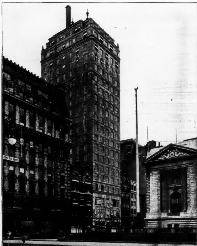
8 West 40th St., New York. Starrett & Van Vleck, Architects. Kewanee Water Heating Garbage Burner installed by Baker, Smith & Company
