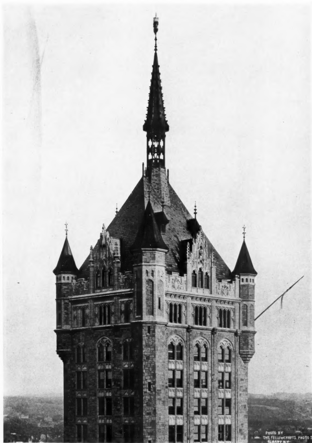
UPPER DETAIL OF TOWER
