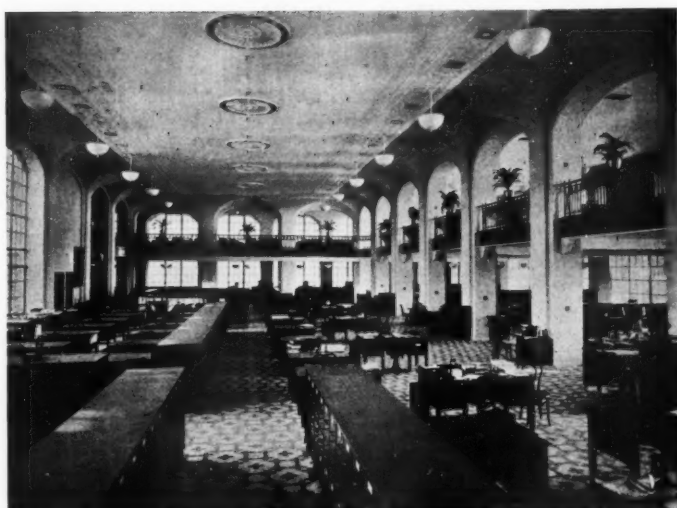
AN OFFICE FLOOR IN THE HILL BUILDING, NEW YORK MESSRS. STARRETT & VAN VLECK, ARCHITECTS
