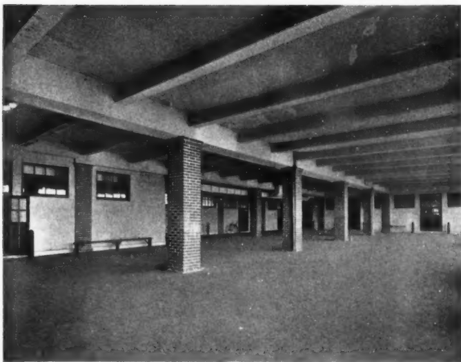
BASEMENT, McCHESNEY SCHOOL
