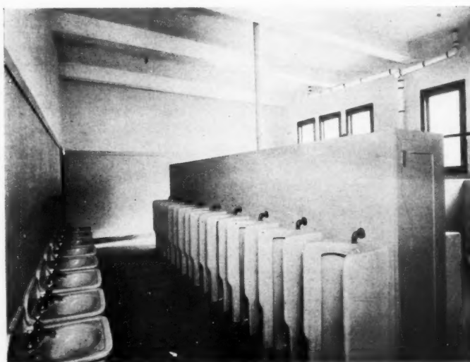
TYPICAL BOYS' TOILET ROOM, DURANT SCHOOL
