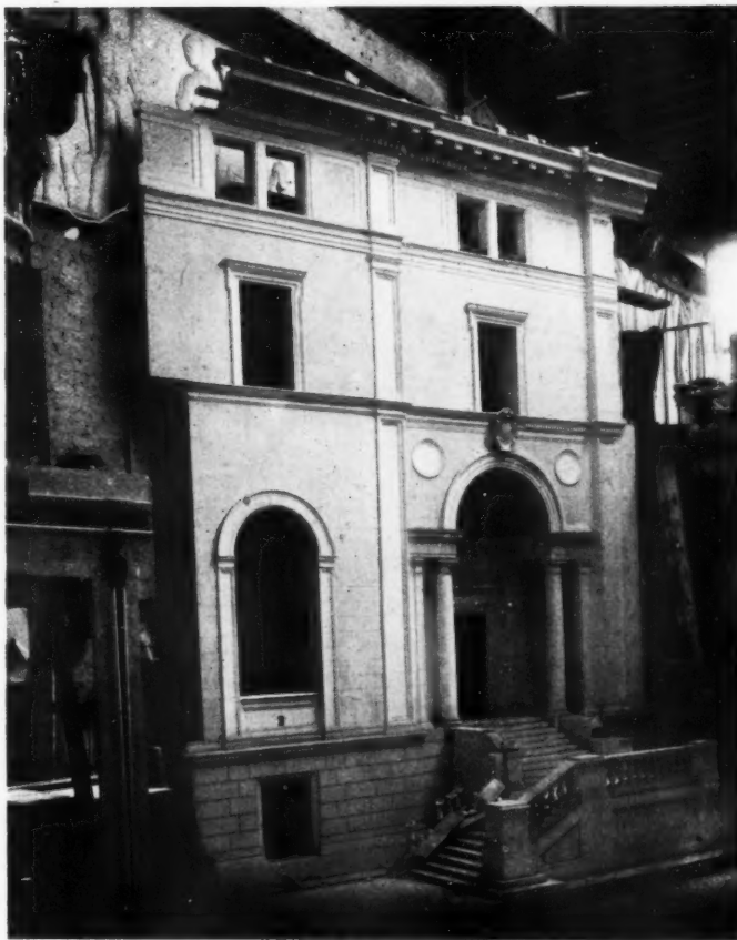
THREE-INCH SCALE MODEL OF A FACADE MR. ELECTUS D. LITCHFIELD, ARCHITECT
