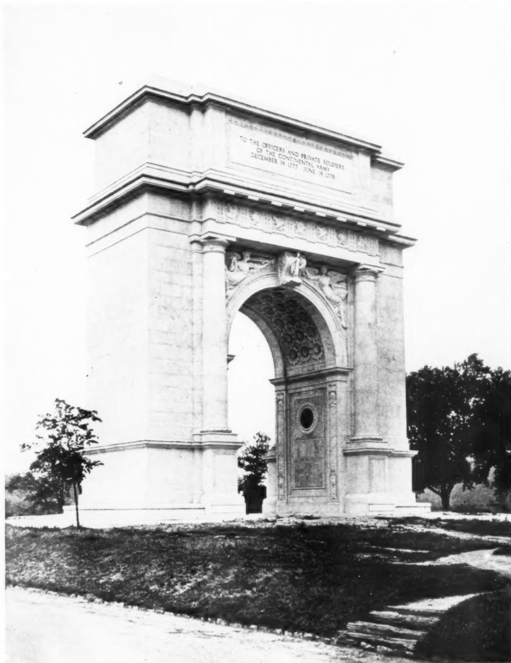
MEMORIAL ARCH AT VALLEY FORGE, PA.
