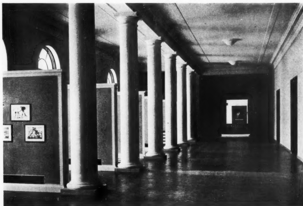
SECOND FLOOR CORRIDOR
