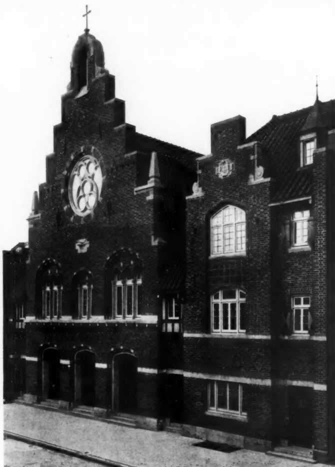
CHURCH OF ST. GEORGE AND RECTORY, BROOKLYN, N. Y. McDERMOTT & HANIGAN, BUILDERS R. J. REILEY, ARCHITECT Hy-tex Falls Creek Velours, full range, laid in \frac{5}{8} inch mortar-joint, rough, cut flush, and limestone colored.
