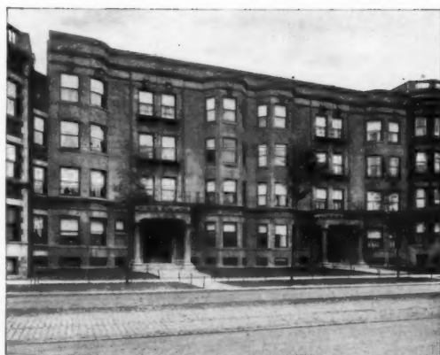
16 Apartment Building at No. 1047 E. 47th St. Chicago. Kewanee Garbage Burner installed.
