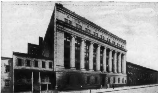
Regis School, New York, N. Y. Meginnis & Walsh, Architects, Boston. Kewanee Smokeless Boilers Installed
