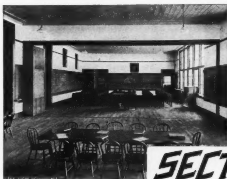
Partition Folded: Note the unobstruc- ted view and the absence of posts.
