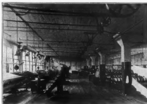
Interior, Showing Corr-Plate Floor.
