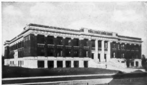
Champaign High School, Champaign, Illinois Spencer & Temple, Arch., Champaign. Kewanee Smokeless Boilers Installed
