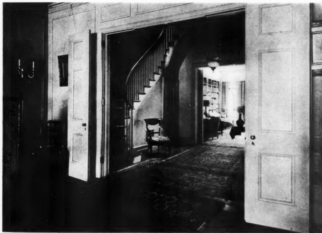
DINING ROOM AND STAIR HALL
