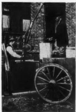
Residence of GEORGE MCKESSON BROWN Huntington, L.I. CLARENCE LUCE, Architect TWO G&G Telescopic Hoists in use
