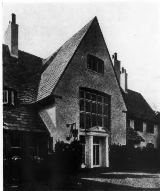
DETAIL OF A HOUSE AT CONVENT, N. J. MESSRS. ALBRO & LINDBERG, ARCHITECTS
