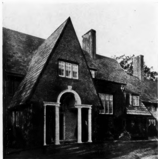
DETAIL, HOUSE AT MORRISTOWN, N. J. MESSRS. ALBRO & LINDBERG, ARCHITECTS
