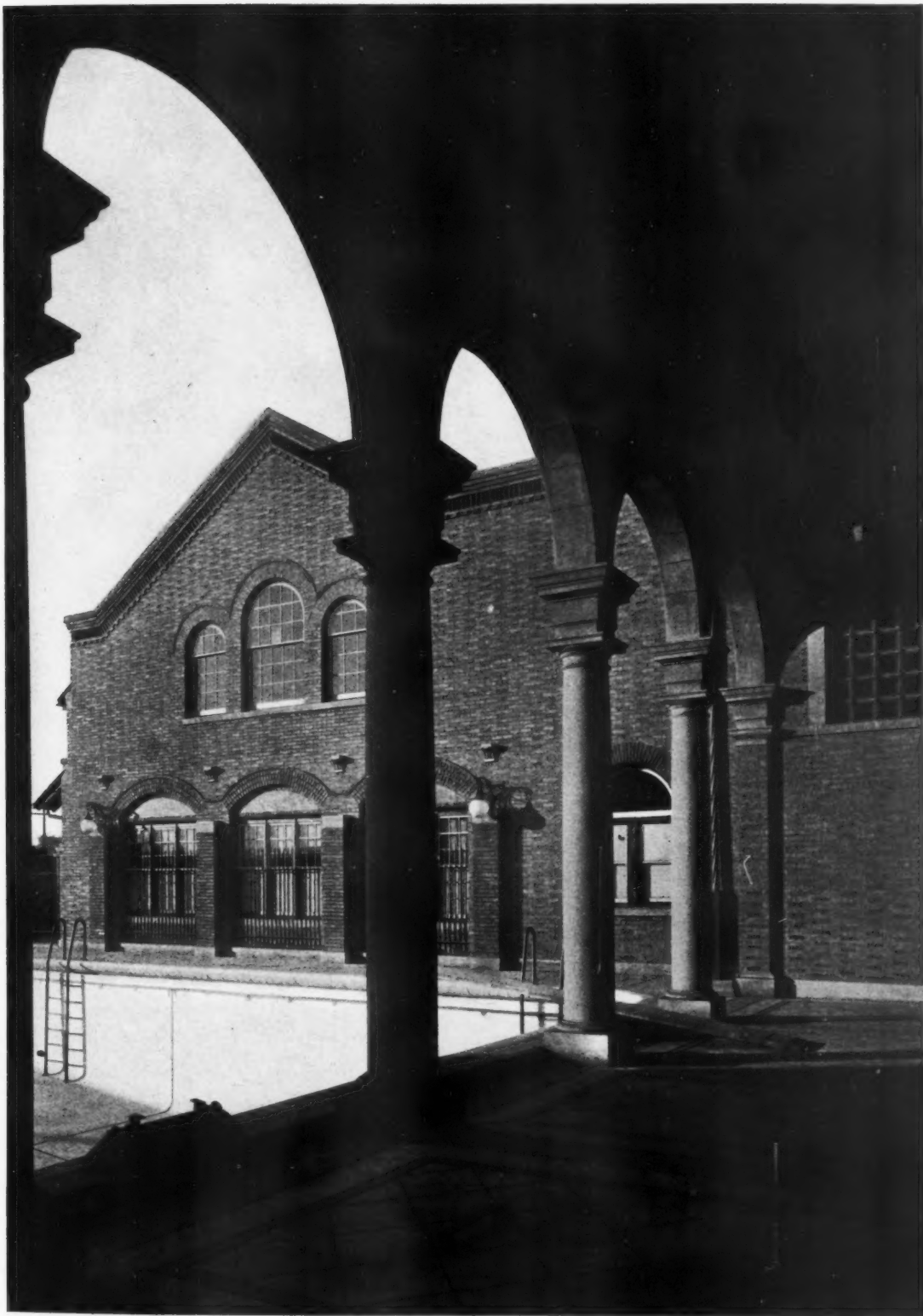
SWIMMING POOL LOGGIA
