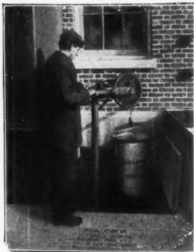
In operation—Raising 200-lb. load of ashes with only 14-lb. pressure on hoisting handle.
