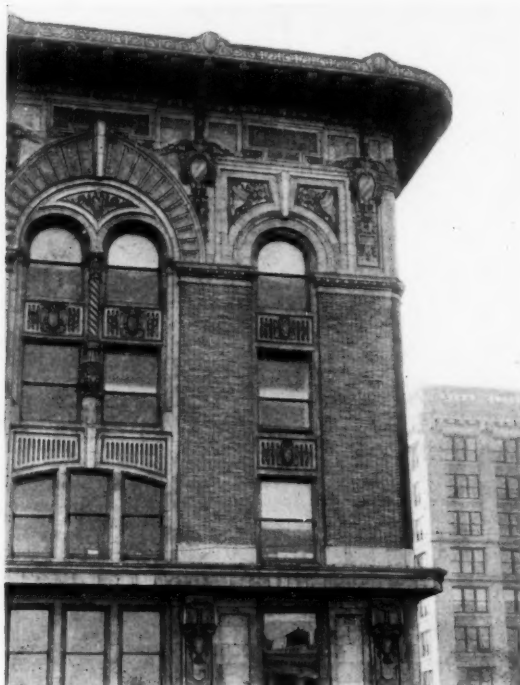
FIG. 20—CORNICE, FOURTH AVENUE BUILDING MR. CHARLES A. VALENTINE, ARCHITECT
