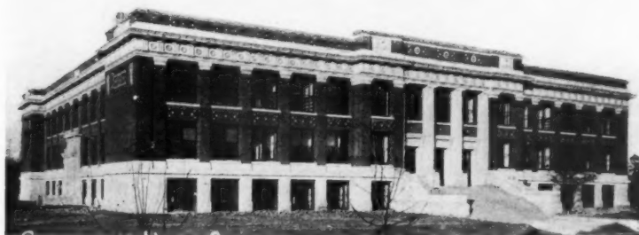
CHAMPAIGN HIGH SCHOOL, CHAMPAIGN, ILLS. Spencer & Temple, Champaign, Architects: Carson Payson Co., Danville, Heating Contractors. Two No. 120 Kewanee Smokeless Firebox Boilers installed.
