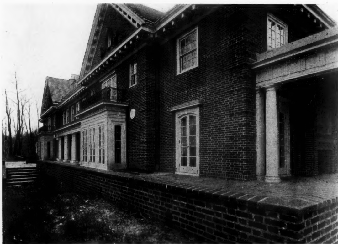
HOUSE ON AN ESTATE AT HUNTINGTON, L. I., NEW YORK
