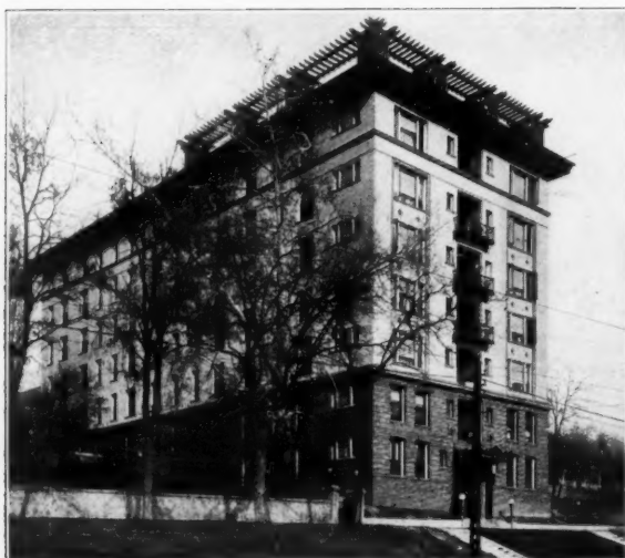
Covey Apartments, Salt Lake City. D. C. Dart, Architect, Salt Lake City.
