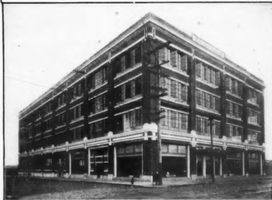
Ford Motor Co., Columbus, Ohio. United Steel Sash used in Windows.
