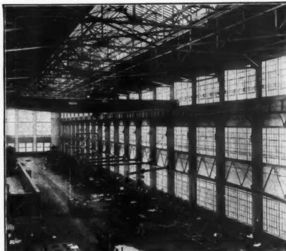
Erecting Shop, The Industrial Works, Bay City, Mich. Albert Kahn, Architect; Ernest Wilby, Associate. Windows of United Steel Sash. Sidings are of concrete plastered on Hy-Rib.
