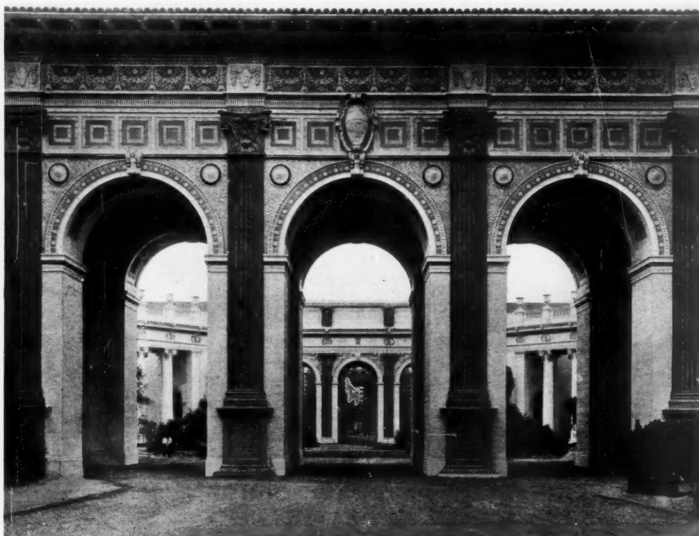
DETAIL OF ARCH, LOOKING TOWARDS COURT OF FOUR SEASONS
