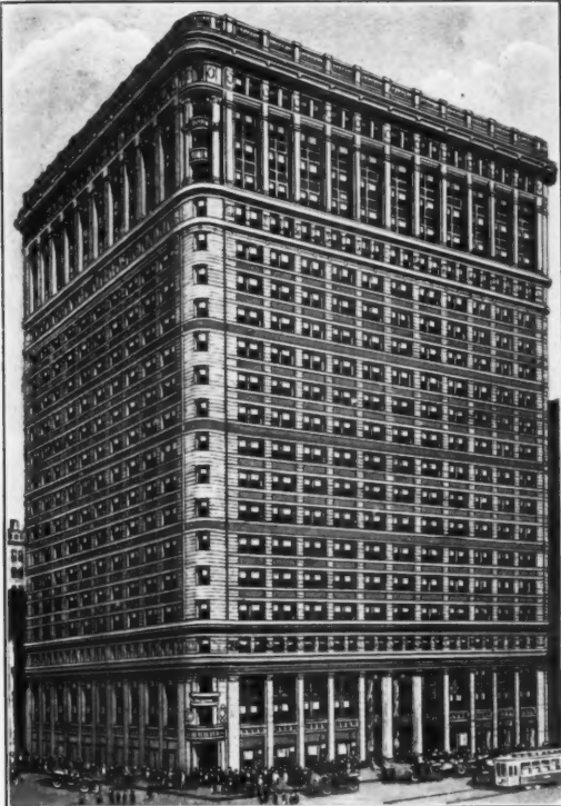
CONWAY BUILDING, CHICAGO Graham, Burnham & Co., Architects F. E. Newberry Elec. Co., Electrical Contractor
