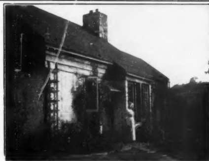
Residence of J. Acker Hays, architect. Stucco stained with Cabot's Stucco Stains "I used your White Waterproof Stain with great success." —J. Acker Hays.
