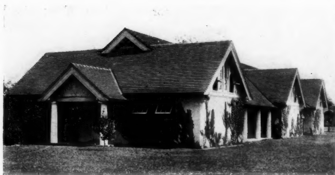
FIELD-HOUSE, GLENFIELD PARK, MONTCLAIR, N. J.
