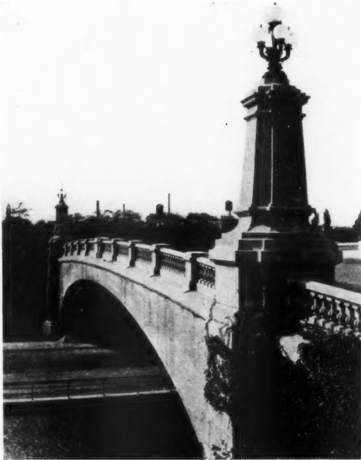
PARK AVENUE BRIDGE, BRANCH BROOK PARK. MR. WALTER COOK, ARCHITECT
