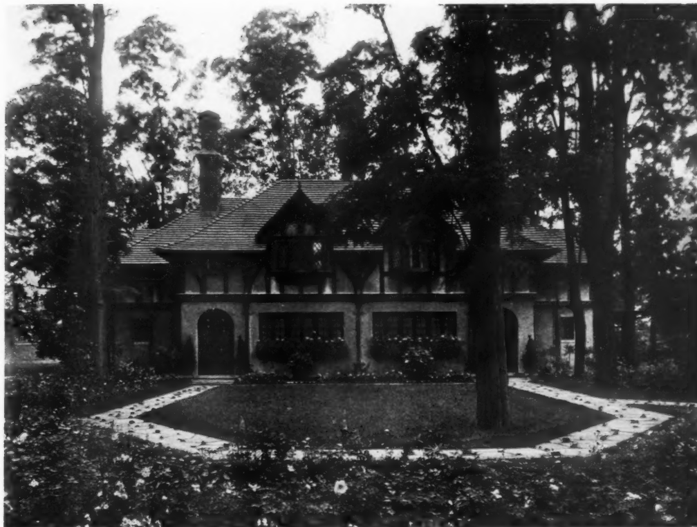
GROUP C—COTTAGE ON J. E. ALDRED ESTATE
