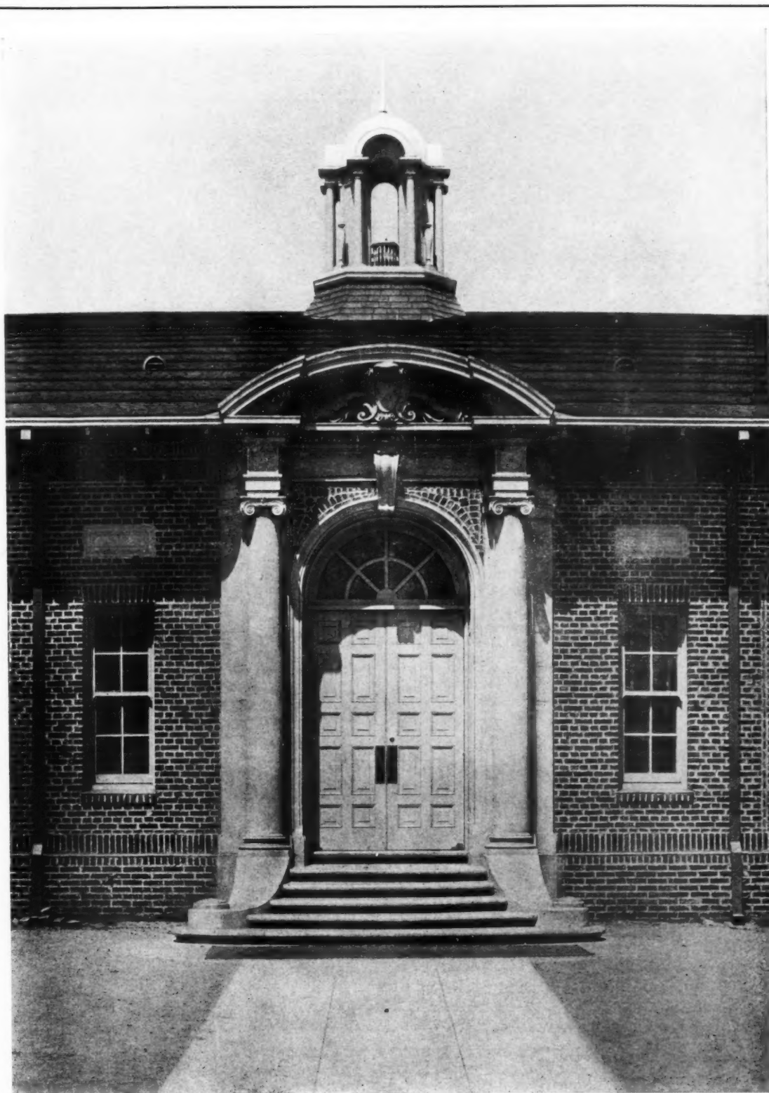
DETAIL OF MAIN ENTRANCE
