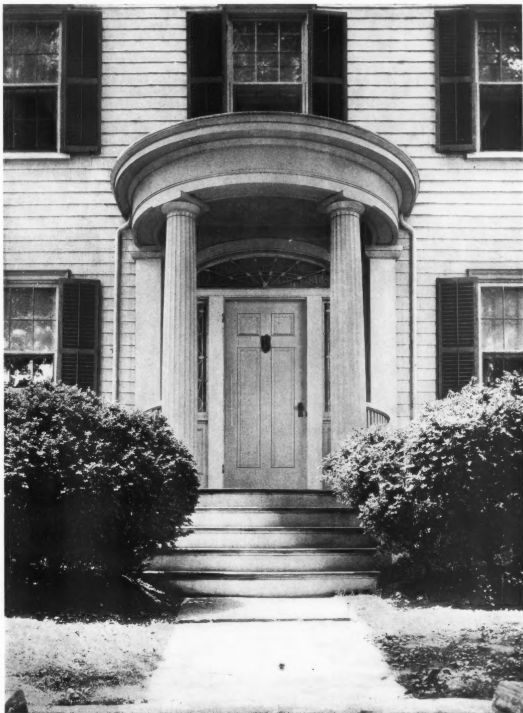
ENTRANCE PORCH AND DOORWAY
