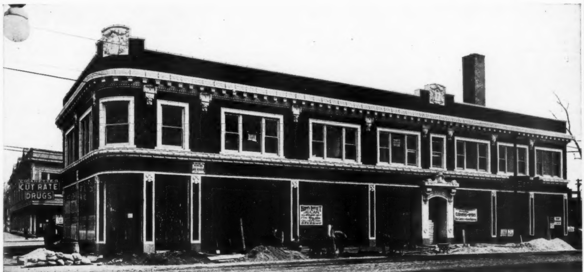
CONSTRUCTION PHOTO OF BUILDING IN CHICAGO TRIMMED WITH MIDLAND T. C.
