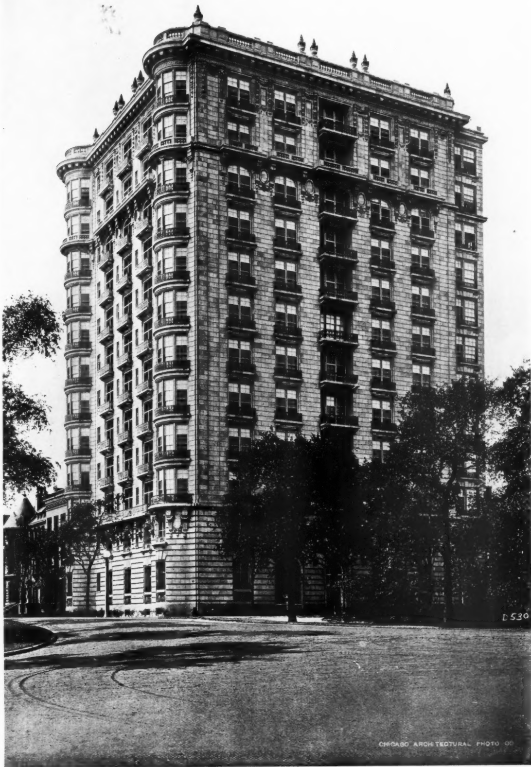
APARTMENT HOUSE, 1550 NORTH STATE PARKWAY, CHICAGO, ILL.
