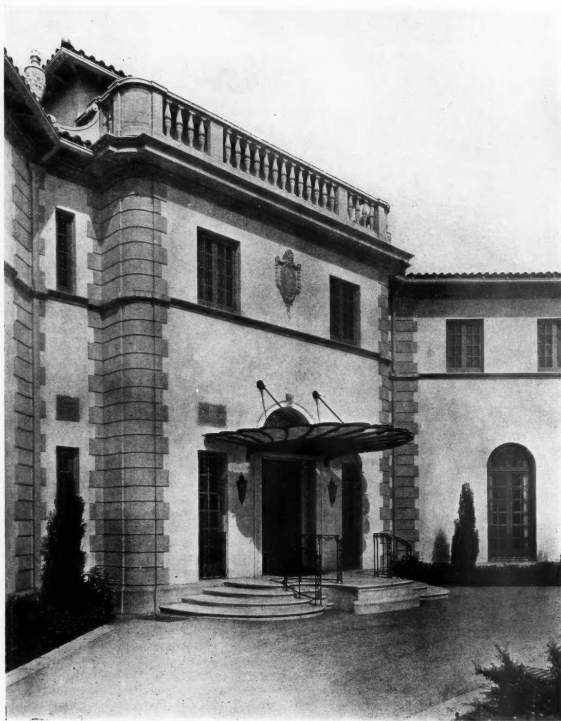
DETAIL OF ENTRANCE
