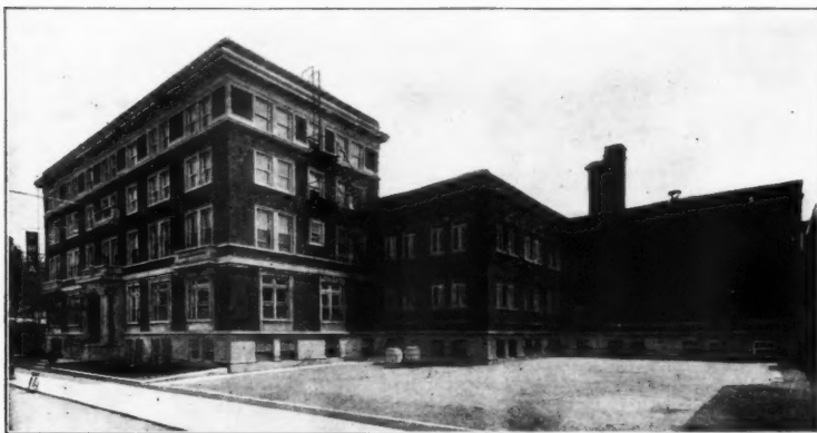
Y. M. C. A. Muncie, Ind. 2 Kewanee Smokeless Boilers installed
