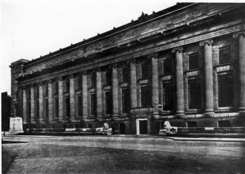
NORTH FACADE—BRITISH MUSEUM EXTENSION
