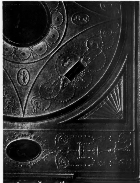
CEILING ON FIRST FLOOR NO. 1 BEDFORD SQUARE, LONDON
