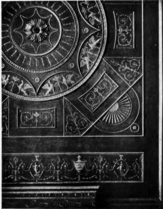
CEILING ON FIRST FLOOR NO 47 BEDFORD SQUARE, LONDON
