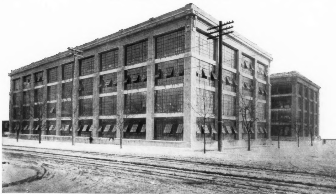
Partial View of the Fenestrated Industrial Buildings
