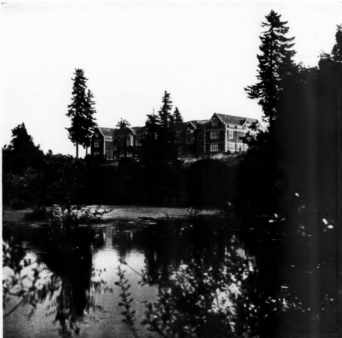
ARTS AND SCIENCE BUILDING
