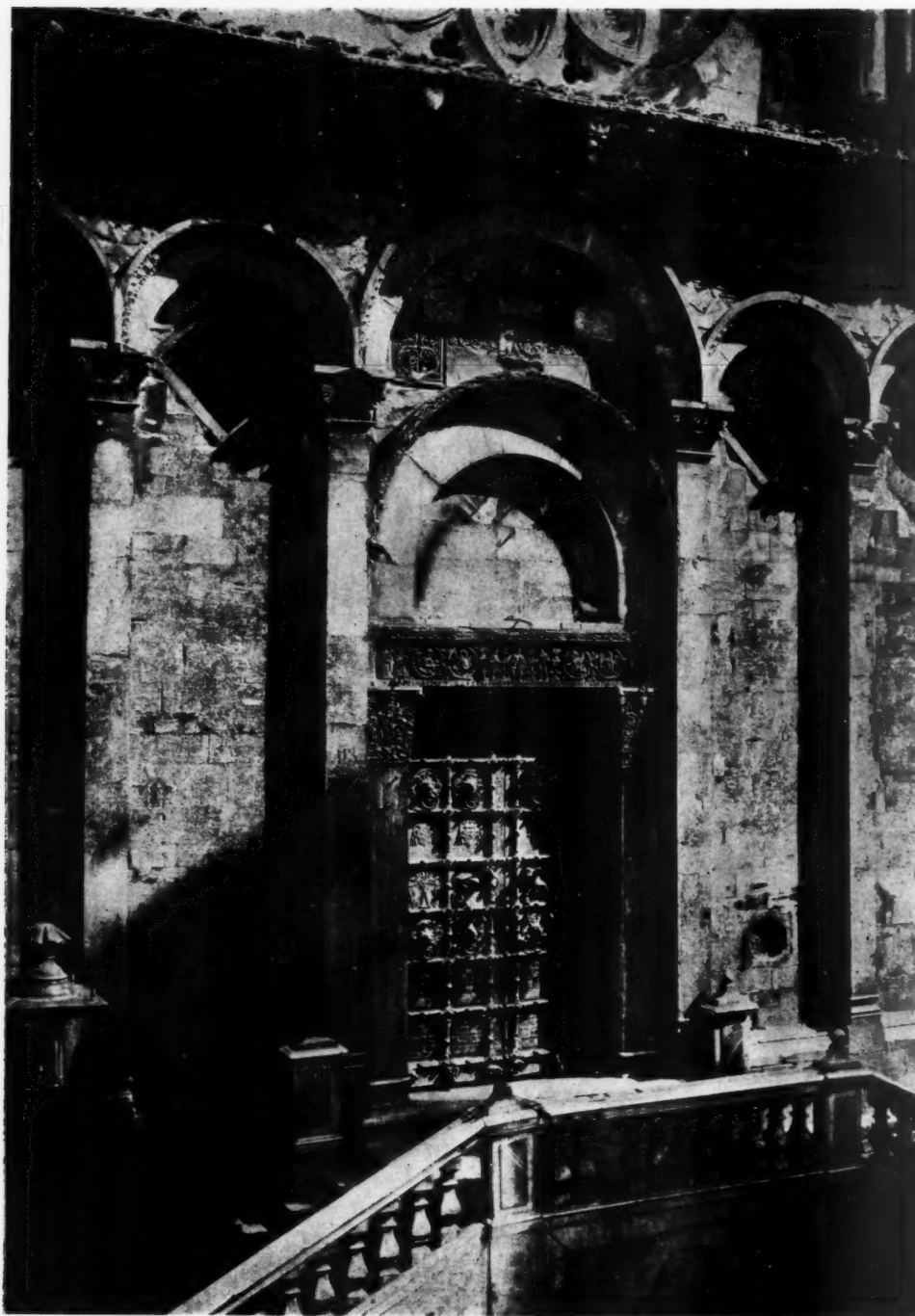
DETAIL OF DOORWAY, CATHEDRAL OF TROIA
