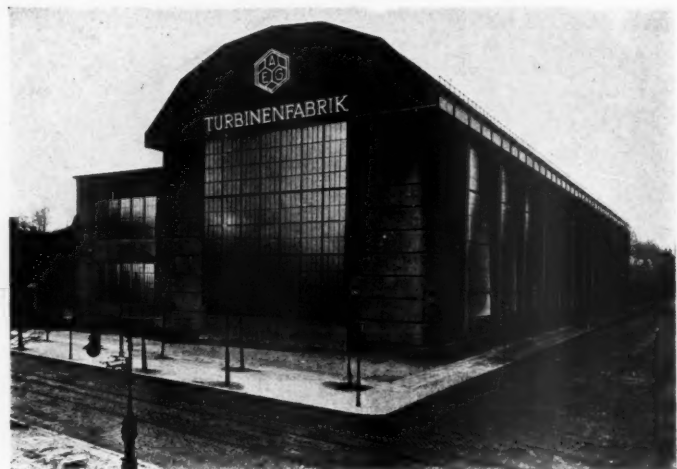
TURBINE ERECTING SHOP OF THE A. E. G., BERLIN PROF. PETER BEHRENS, ARCHITECT
