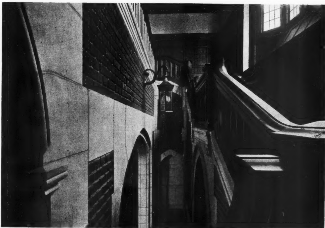
INTERIOR DETAILS, ARTS AND SCIENCE BUILDING REED COLLEGE, PORTLAND, ORE. MESSRS. DOYLE & PATTERSON, ARCHITECTS
