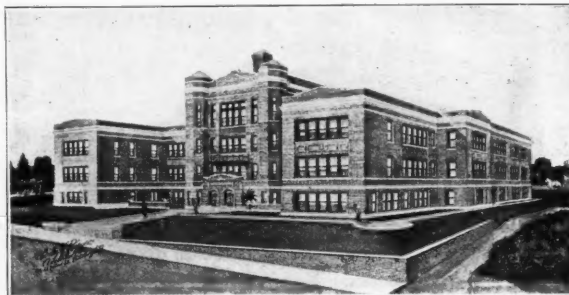
New Kensington High School, New Kensington, Pennsylvania
