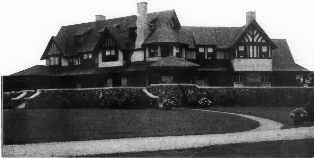
Stucco House of Ex-Governor Eugene N. Foss, at Cohasset, Massachusetts. Erected 1899. Architects, Chapman & Frazer, Boston.
