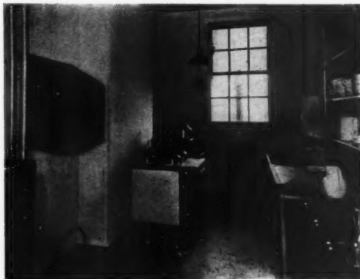
SERVING KITCHEN, WHITE ISOLATION BUILDING
