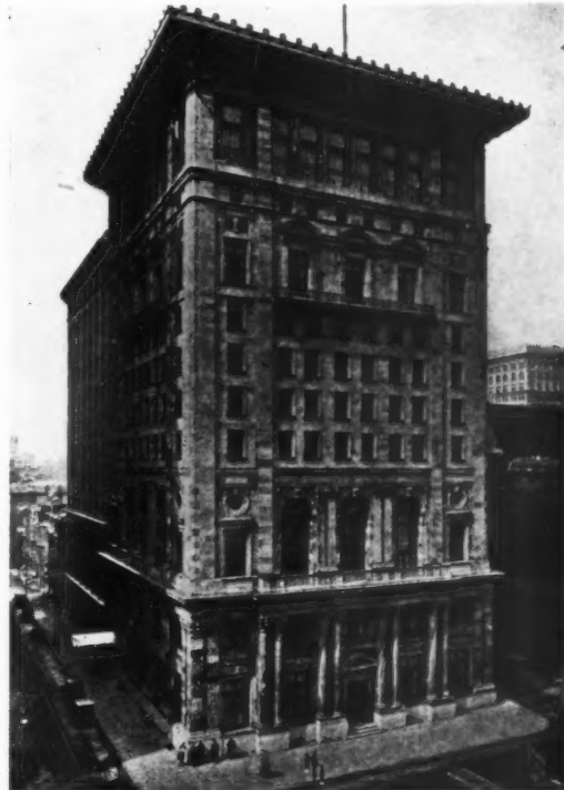
MANUFACTURERS' CLUB, PHILADELPHIA, PA. MESSRS. SIMON & BASSETT, ARCHITECTS
