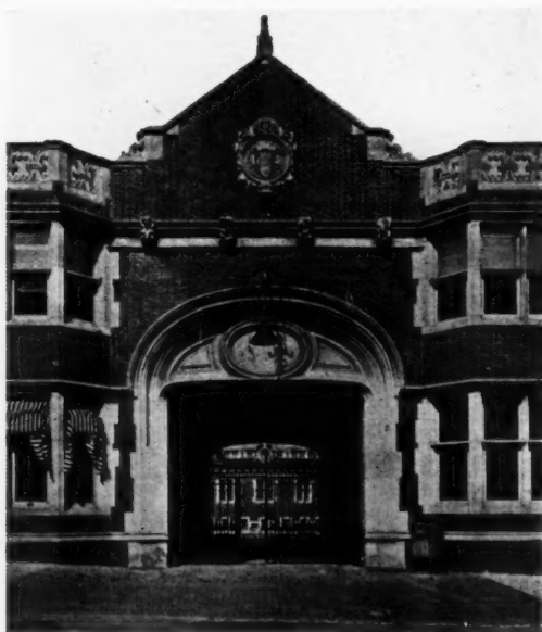
ENTRANCE TO COURT, VETERINARY BUILDING, UNIVERSITY OF PENNSYLVANIA MESSRS. COPE & STEWARDSON, ARCHITECTS
