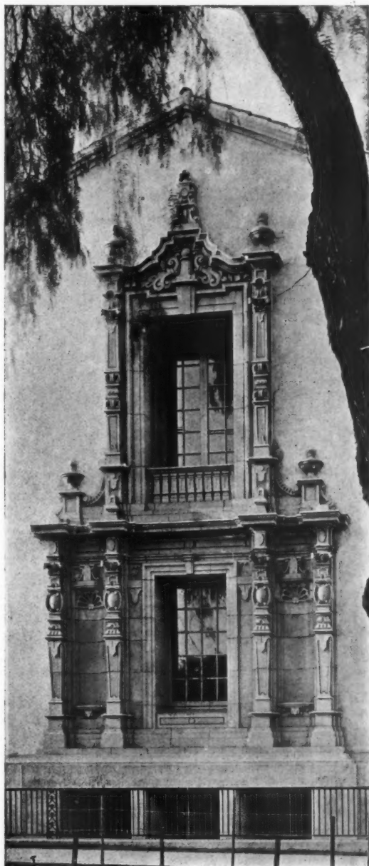
NORTH TRANSEPT WINDOWS
