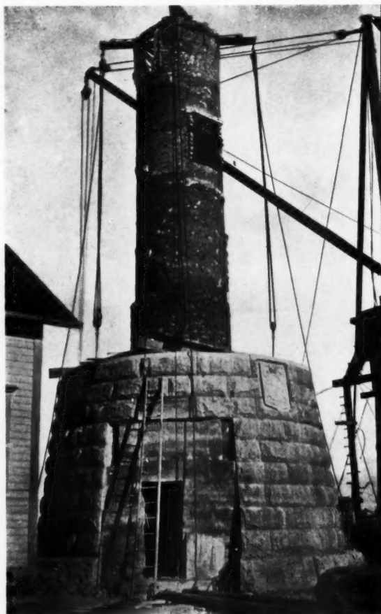
BRICK STAIRCASE OF OLD TOWER, WITH OLD MASONRY REMOVED. SHOWS BASE OF NEW TOWER BUILT AROUND IT
