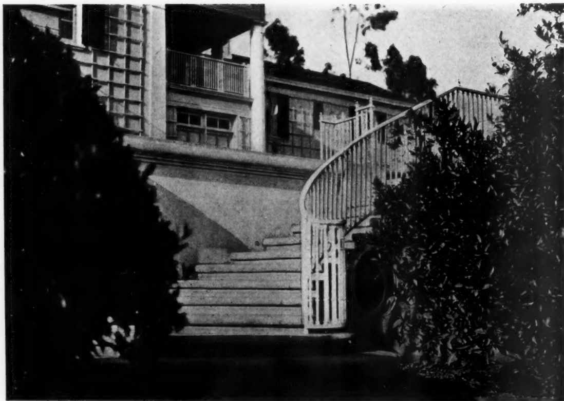
STEPS FROM TERRACE TO GARDEN
