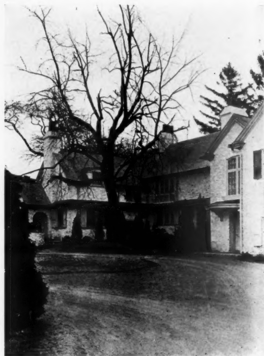
ENTRANCE COURT RESIDENCE AT PAOLI, PA. MESSRS. EVANS & WARNER, ARCHITECTS
