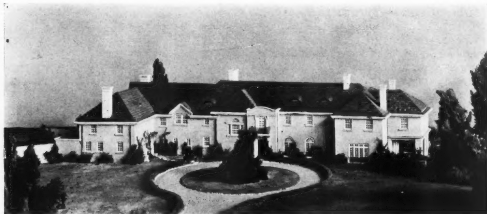
ENTRANCE FRONT—FROM MODEL HOUSE FOR JOHN R. FELL, ESQ., CAMP HILL, PA. MESSRS. STEWARDSON & PAGE, ARCHITECTS
