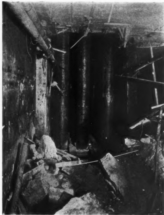
THE PILES ARE MAINTAINED IN A VERTICAL POSITION BY MEANS OF WEDGES APPLIED NEAR THE GROUND LEVEL
