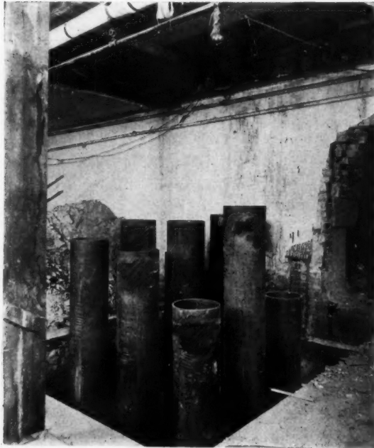
AFTER THE TOPS ARE CUT TO A COMMON LEVEL BY THE OXY-ACETYLENE TORCH, THE PILES ARE REINFORCED WITH TWO-INCH STEEL RODS AND FILLED WITH CONCRETE
