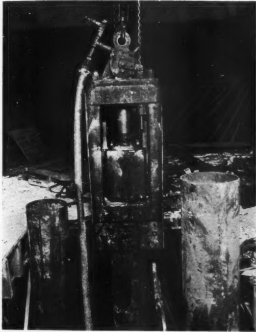
A 3,000-POUND STEAM HAMMER DRIVES THE STEEL SHELLS THROUGH ALL OBSTRUCTIONS TO HARD BED ROCK
