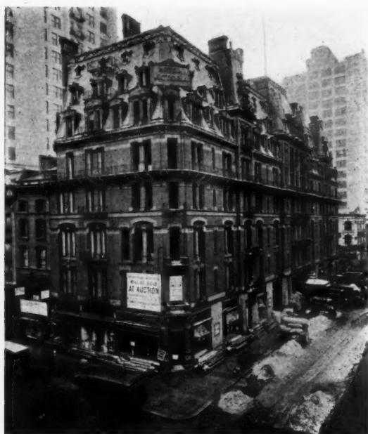
BEFORE THE OLD STRUCTURE WAS VACATED, FOUNDATIONS WERE BEING PREPARED FOR A LOFT BUILDING ON THE SAME SITE
