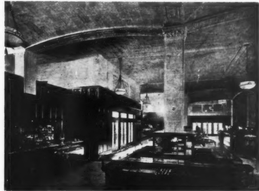
MAIN FLOOR, DEPARTMENT STORE OF LORD & TAYLOR, FIFTH AVENUE, NEW YORK MESSRS. STARRETT & VAN VLEEK, ARCHITECTS (Copyright, Johnston-Hewitt)
