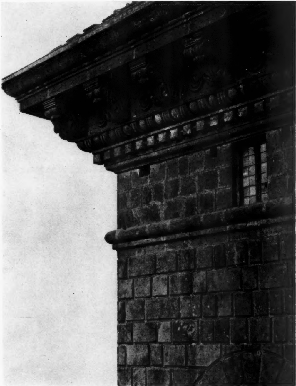
DETAIL OF CORNICE, PICCOLOMINI PALACE, SIENA, ITALY
