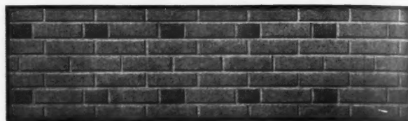
ABOVE—FLEMISH COURSES ALTERNATING WITH TWO COURSES OF STRETCHERS; BELOW—FLEMISH COURSE ALTERNATING WITH THREE ROWS OF STRETCHERS
