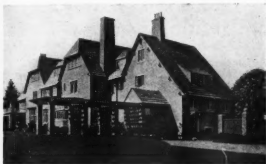
HOUSE AT OYSTER BAY, L. I., N. Y. MESSRS. STEPHENSON & WHEELER, ARCHITECTS
