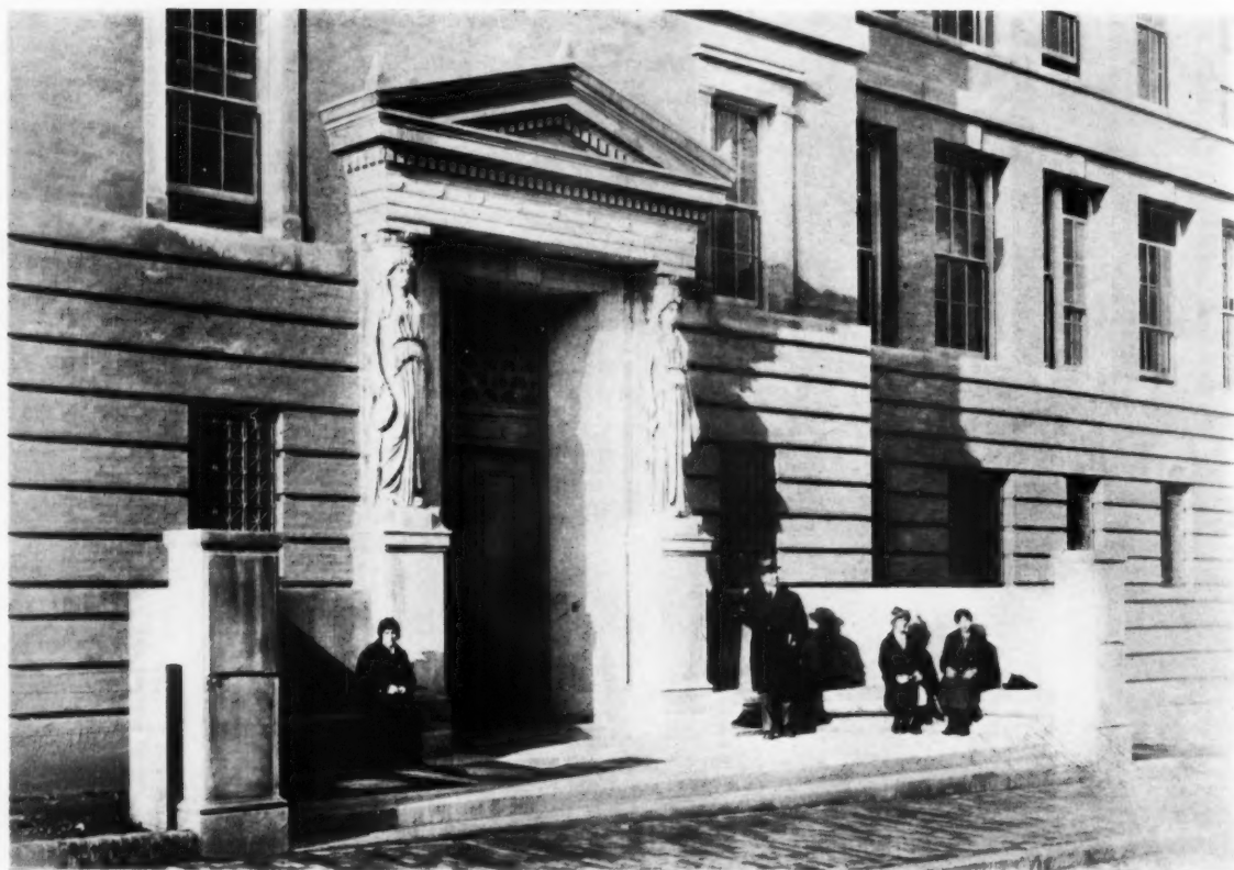
DETAIL OF MAIN ENTRANCE
