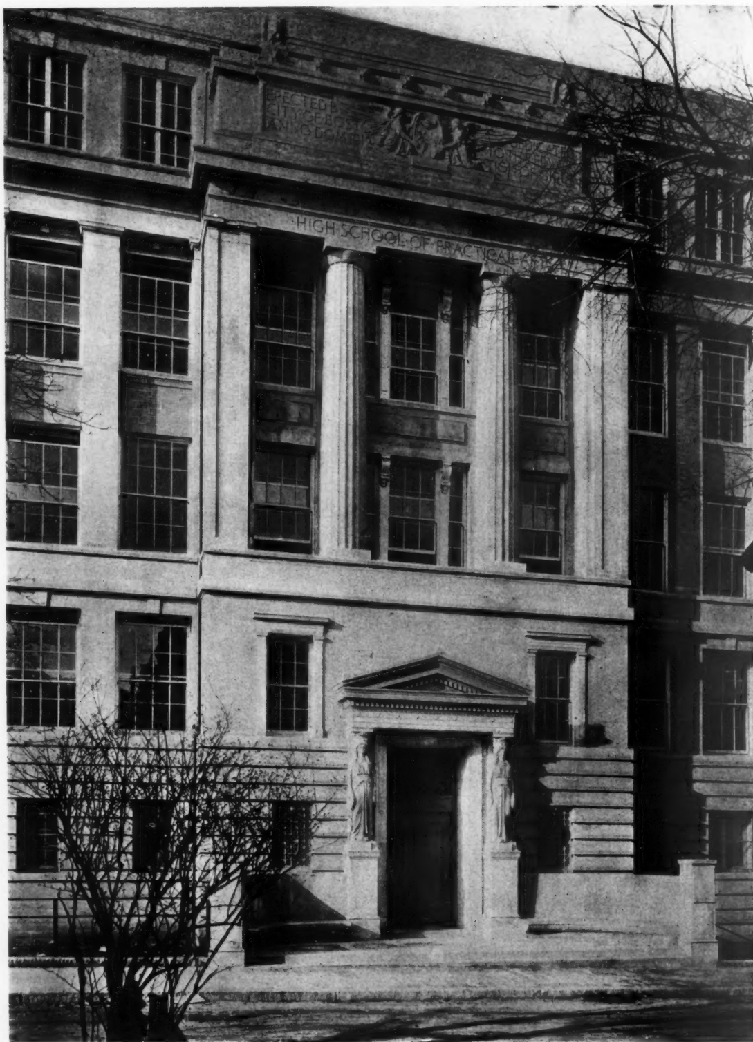
DETAIL FRONT FACADE
