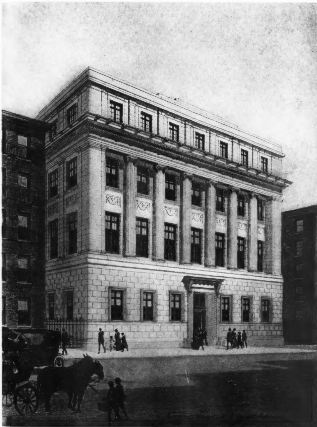
CHILDREN'S COURT BUILDING, 137 EAST 22 D STREET, NEW YORK
