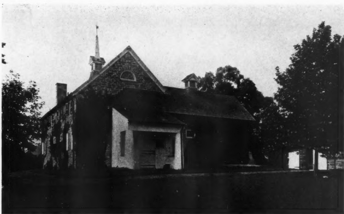
VIEW OF STABLE AND GARAGE, SHOWING COW STABLE
