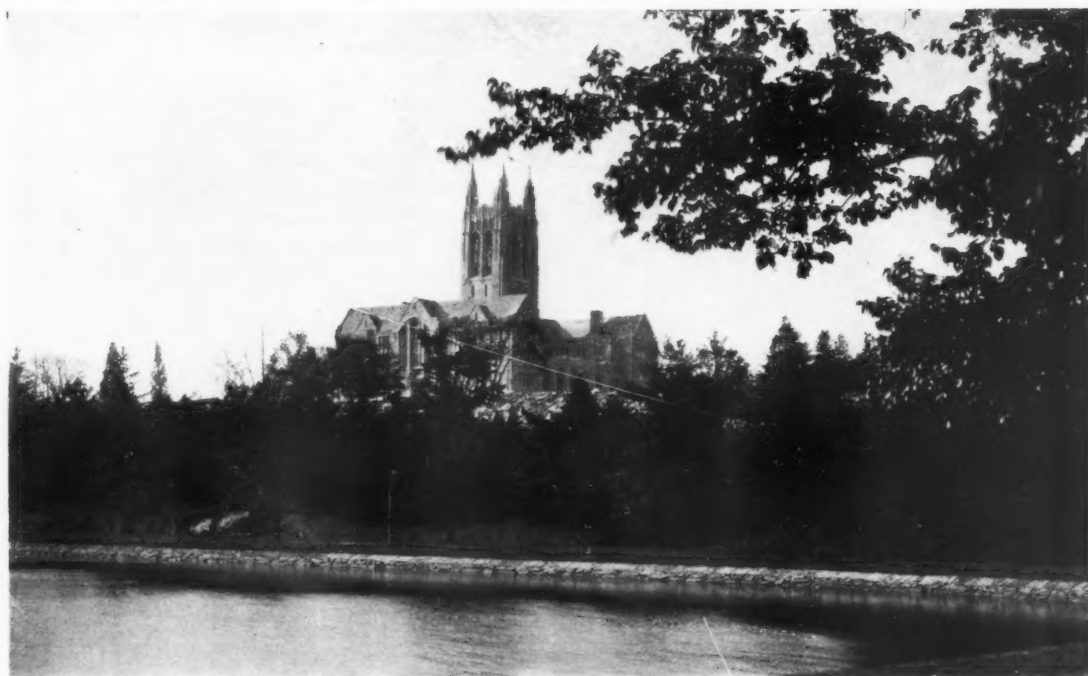
VIEW LOOKING SOUTHWEST
