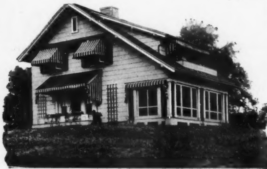
Stained with Dexter Stains Waite & Copeland, Architects, Boston
