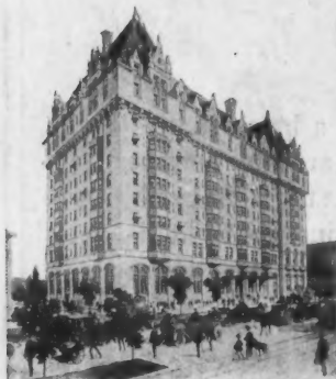
705 Sylphon Packless Valves used in Fort Gary Hotel, Winnipeg, Can. Ross McFarlane & Rugh, Architects; Cotter Bros., Ltd., Heating Contractors.
