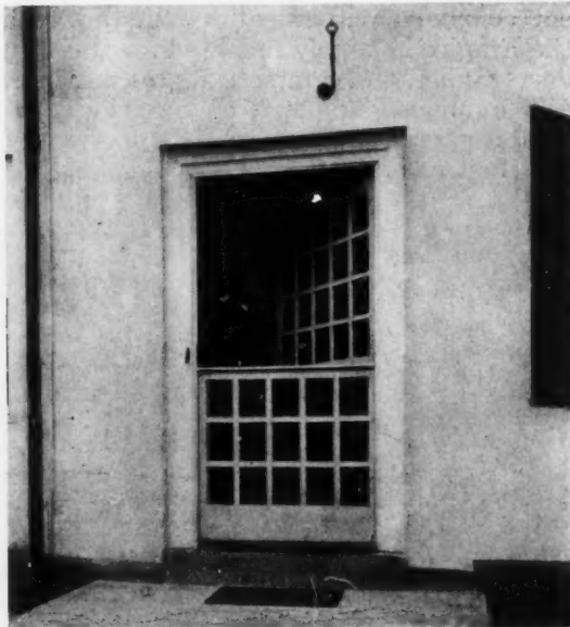
Detail of divided door in Glen House, showing one of the iron numerals used for wall anchors.
