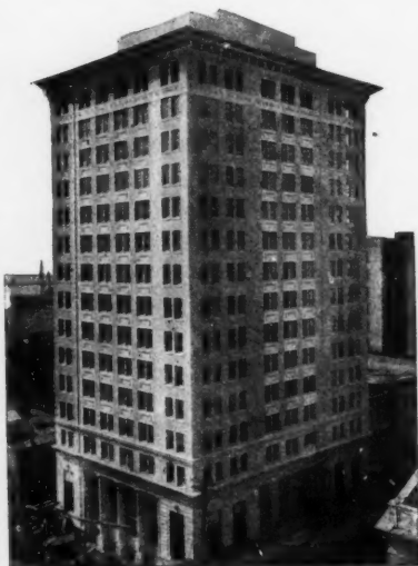
In this splendid office building, the Heard National Bank Building of Jacksonville, Fla., the basement was perfectly waterproofed against ground water by the use of Ceresit. Architect, John Kevan Peebles, Norfolk, Va.
