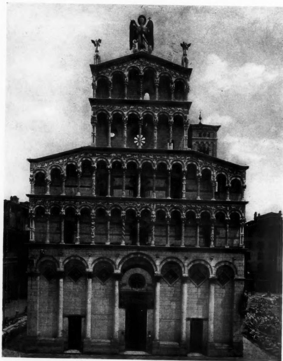
FACADE, CHURCH OF ST. MICHAEL, LUCCA, ITALY
