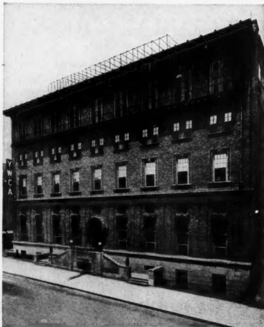
Y. W. C. A. BUILDING, ST. LOUIS, MO. MARINER & LA BEAUME, ARCHITECTS
