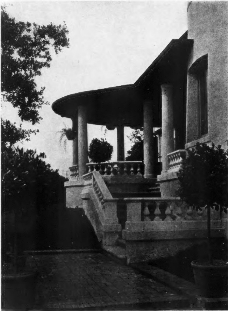
ENTRANCE, HOUSE OF MR. ELMER GREY, OAK KNOLL, PASADENA, CAL. MR. ELMER GREY, ARCHITECT
