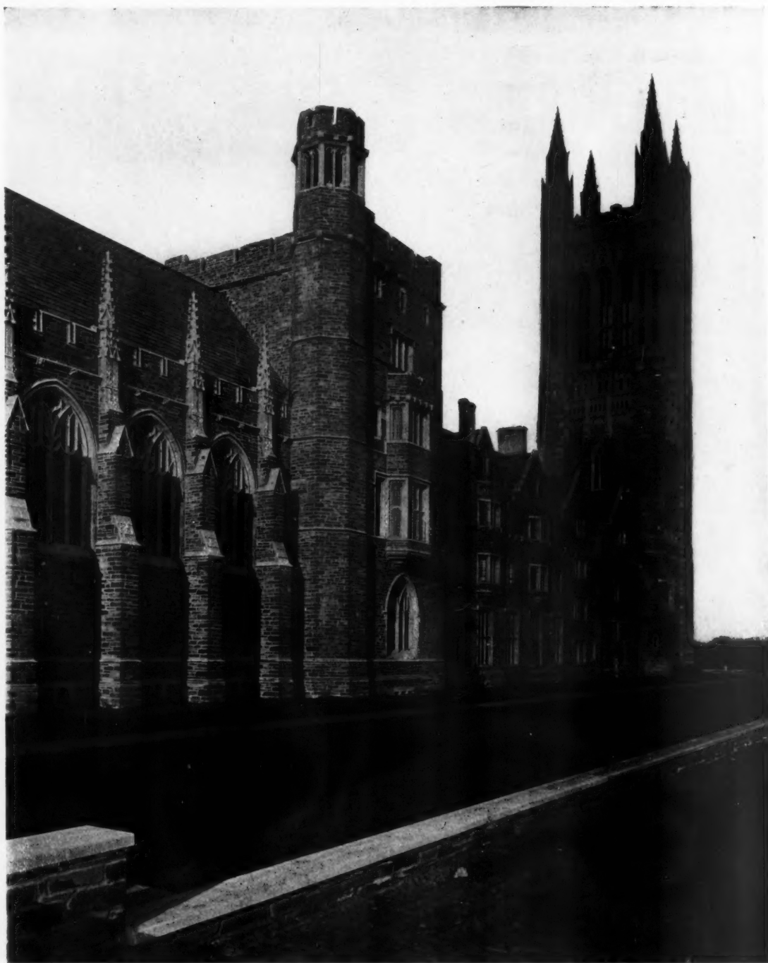
LOOKING ALONG SOUTH ELEVATION
