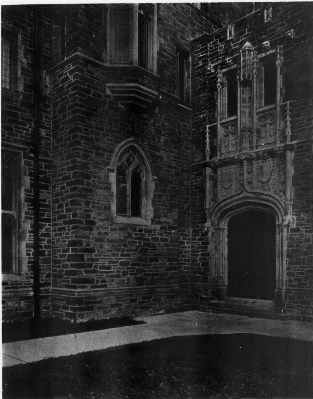
DETAIL OF SOUTHWEST CORNER OF QUADRANGLE
